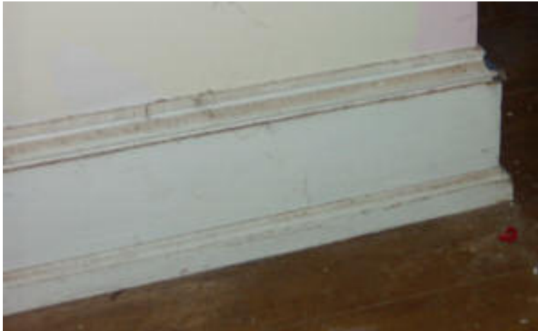
Molding 6. Spiked baseboard molding, found on the second floor of the center section.
