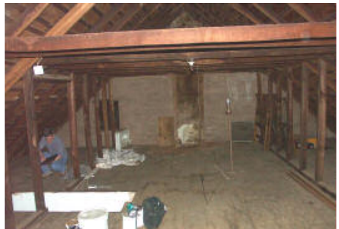
Photo 29. Interior of attic, center section.
