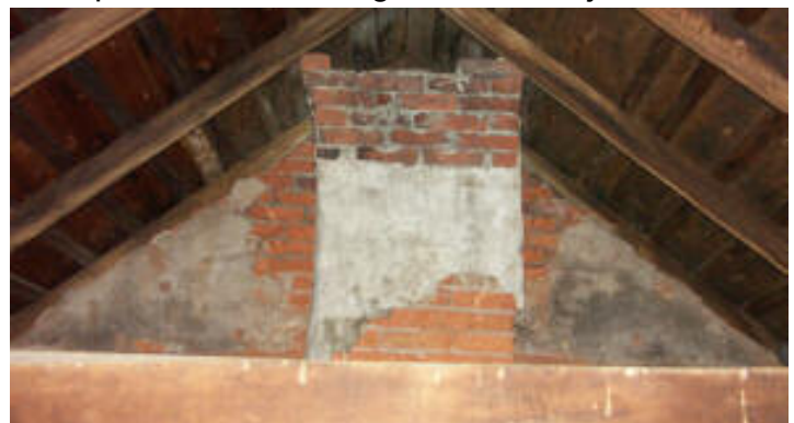
Photo 28. Chimney, south end of main block.
