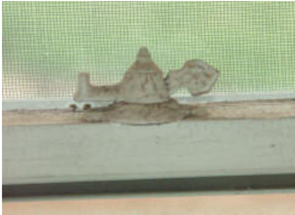
Photo 24. Victorian window latch in Room N4.
