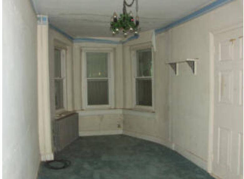
Photo 21. Room C4, center section, facing west into bay window.
