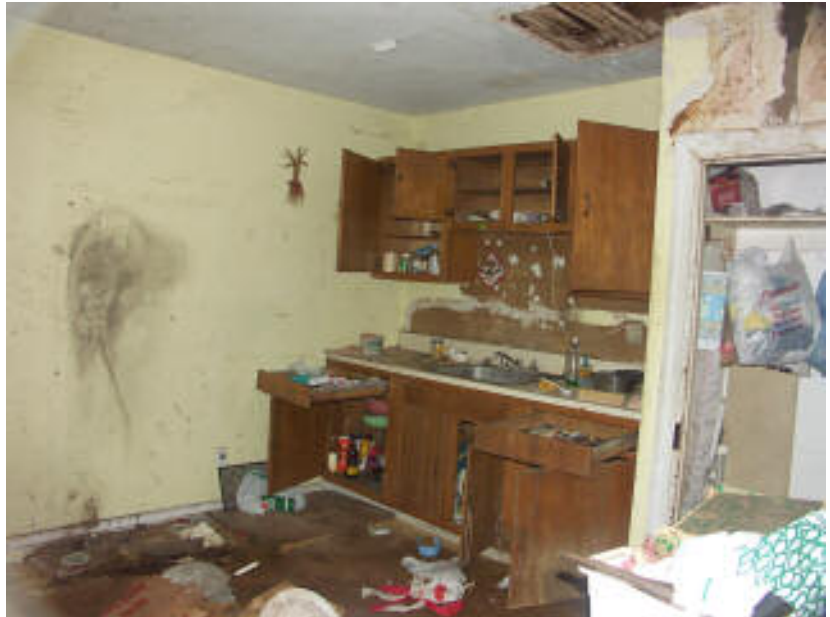
Photo 19. Room C2 in center section, facing NW.
