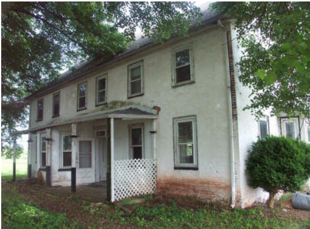
Photo 2. West and part of south elevations of House.
