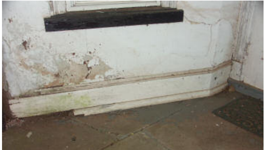
Photo 4. Exterior baseboard molding on porch, west elevation.
