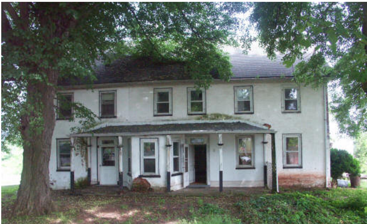
Photo 1. Hunsicker House, west elevation.
