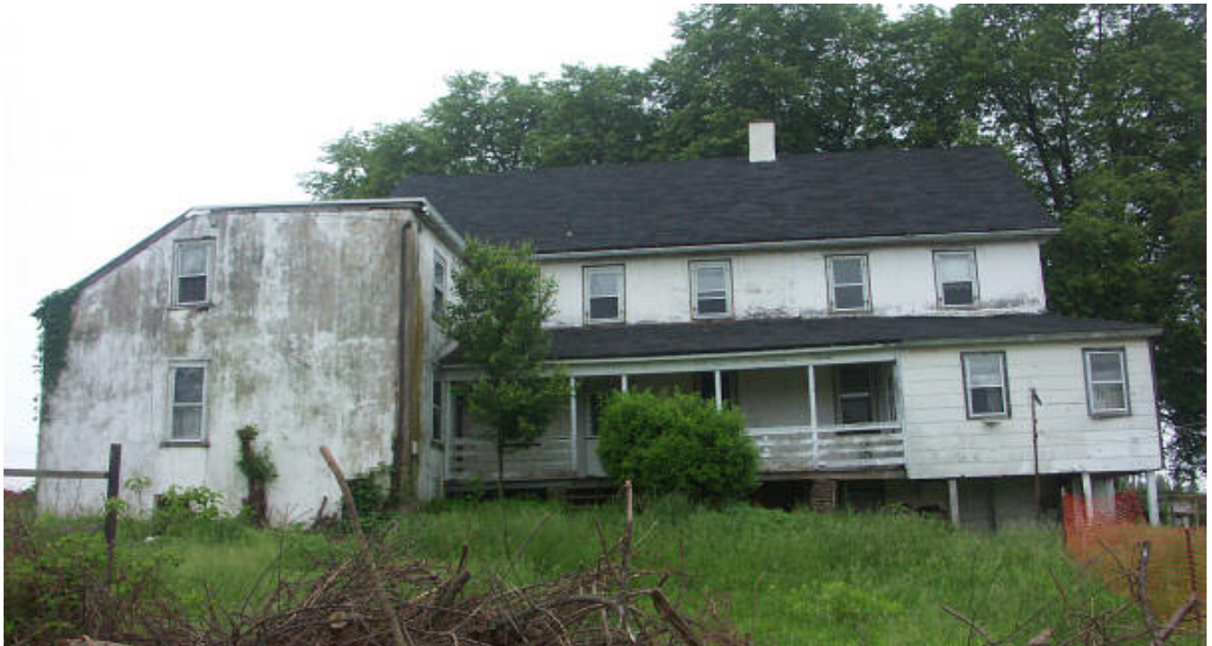
Photo 7. East elevation of House, showing south section (L) and main block (R) .
