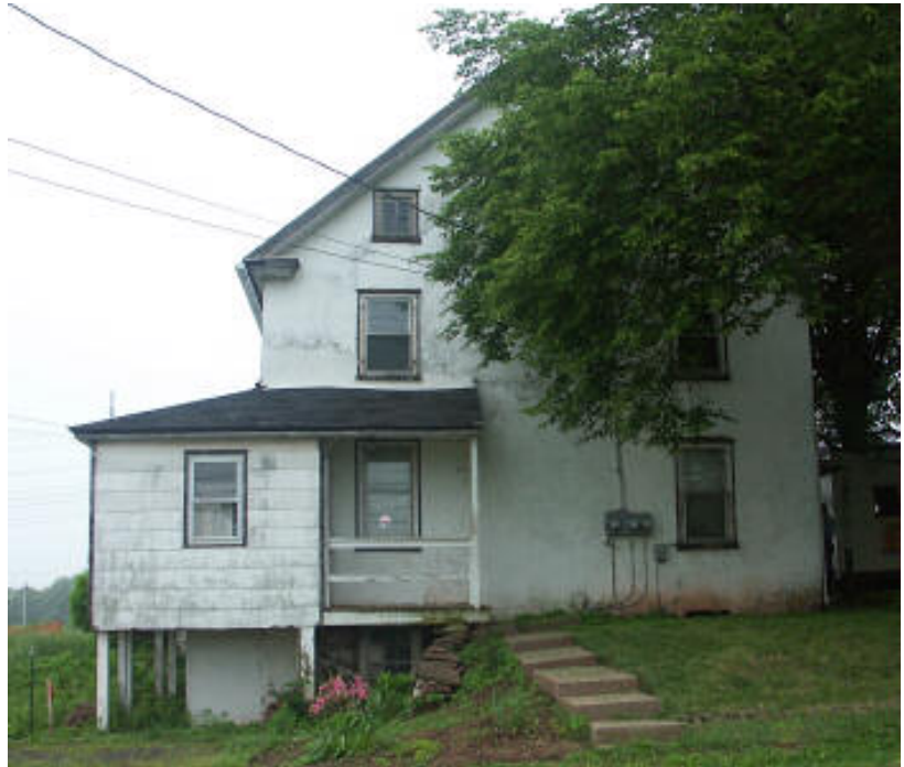
Photo 9. North elevation of House. Frame section on left.
