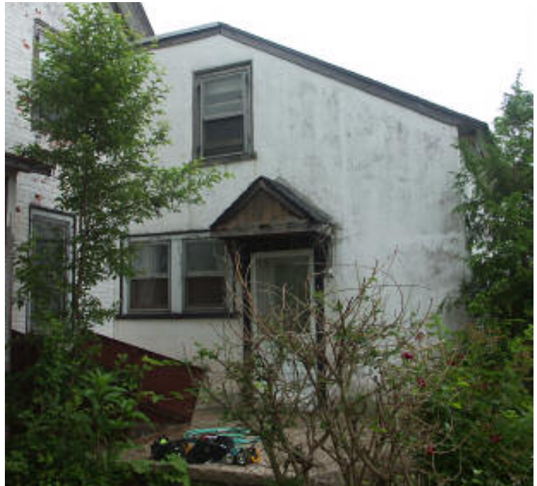
Photo 11. West elevation of south section.
